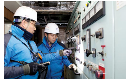
Inspection activities by the Safety Assurance Team at Dongwon Industries
